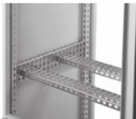
Grid strap installation (from side to side).
